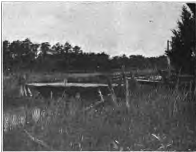
BRIDGE OVER GAMBO CREEK.
